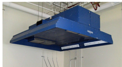
Fume Booth For Grinding, Sanding, Deburring, Painting.
